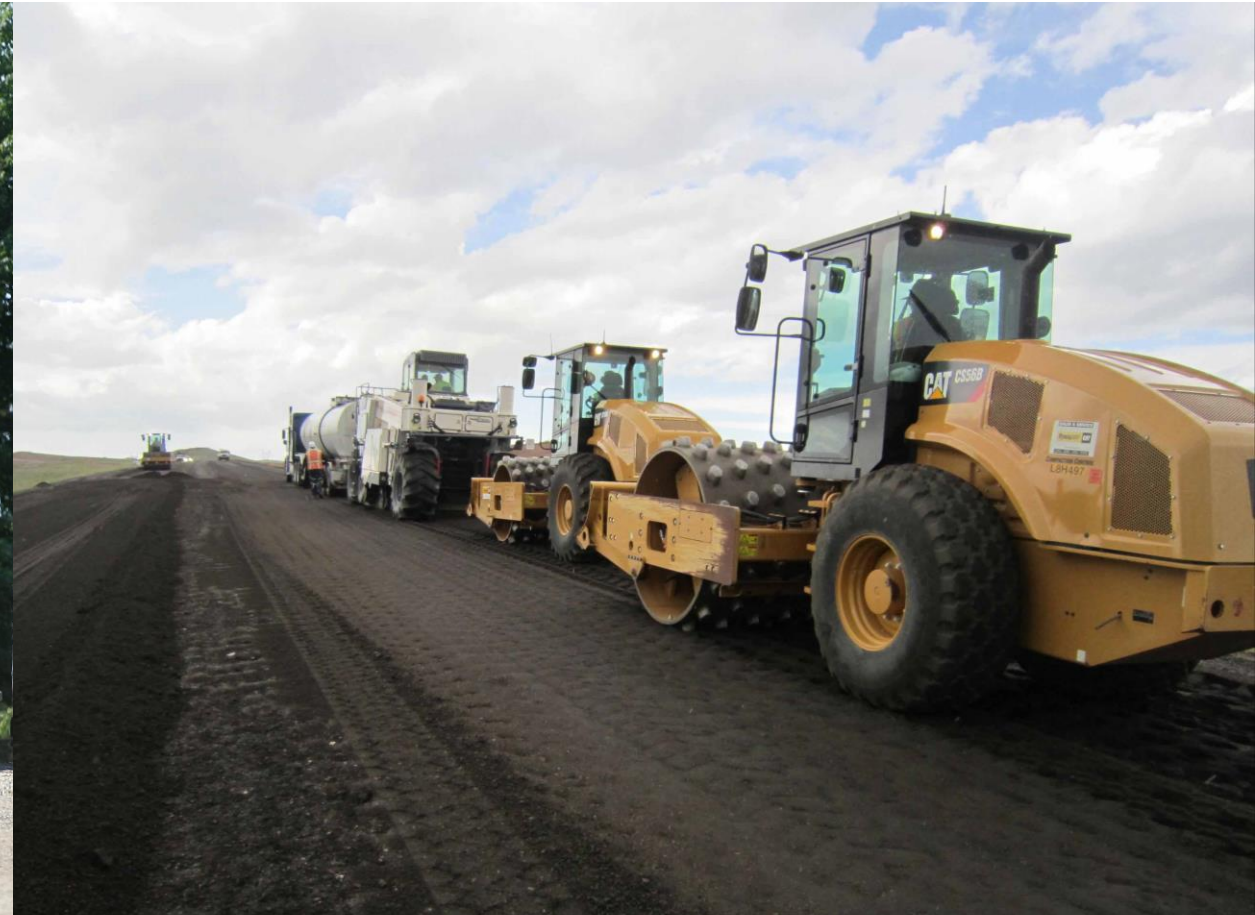
Full Depth Reclamation In-Situ Recycling
