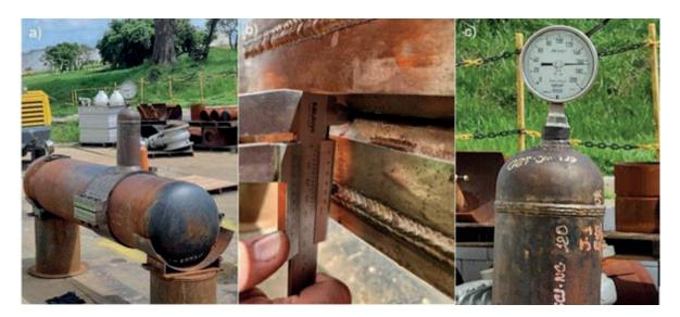
Figure 6 - a) Installed clamp; b) Recording of the flange gap; c) Recording of the achieved pressure.
