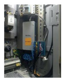
Figure 5 - Data acquisition (DAQ) system installed in the electrical panel.
