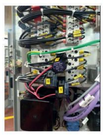
Figure 6 – Current transducers on the power cable and in the induction motor panel.
